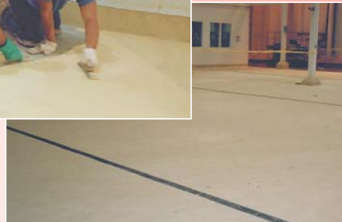
Trowel applied resin systems. Available in different resin components and formulations to suit unique service conditions. These systems yield a durable, chemical resistant floor topping where chemical conditions are less harsh and where traffic conditions are light.
